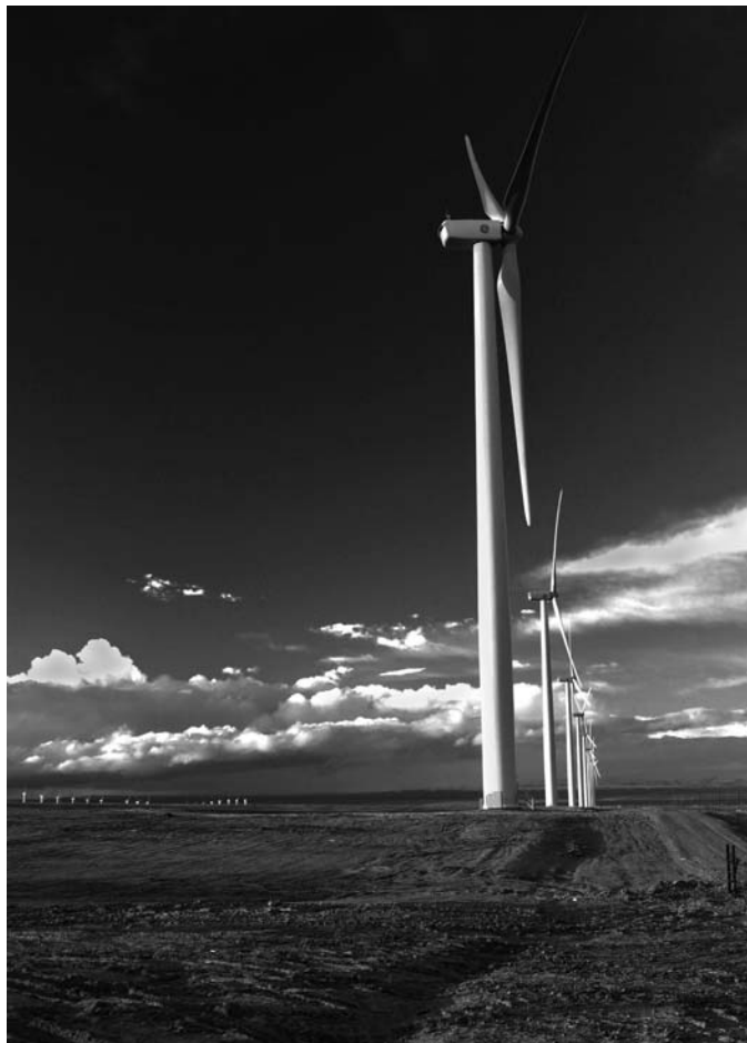
Wind Power Generation
