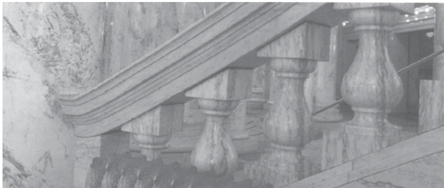
Capitol Interior Stairway
